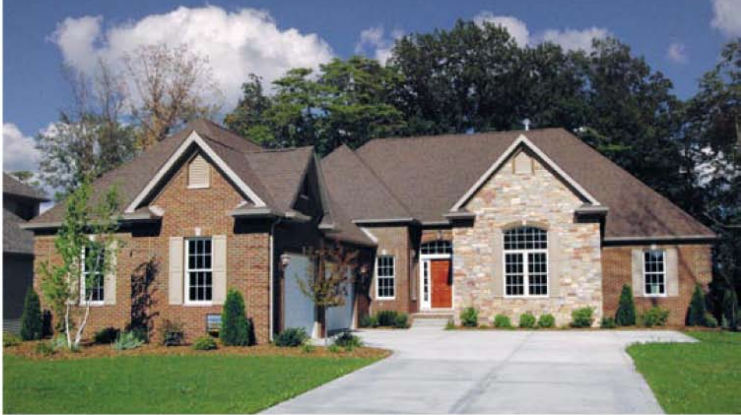
Sommers Construction home built at the Links of Aberdeen.
